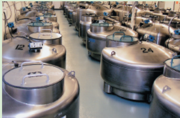
Main liquid nitrogen storage facility at Coriell
